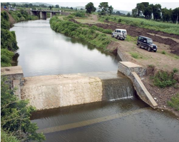
Fig 1: A water conservation system in Shirpur
