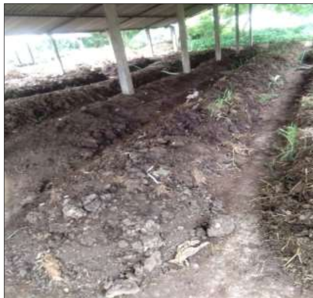
Photo 1: Construction of Vermibeds
